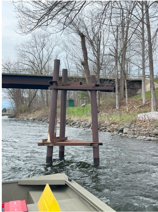
Photograph 9: Large metal structure upstream of Morgan Road.
