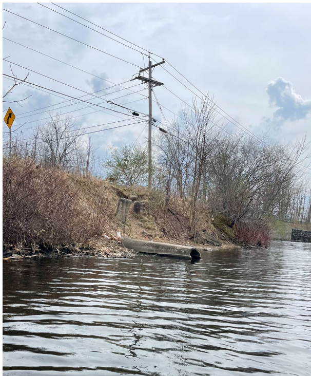
Photograph 4: Diffuser pipe location marked with concrete posts, former concrete outfall pipe.
